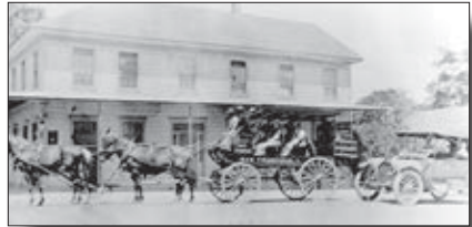
Skaggs Stage from Geyserville Hotel to Skaggs Springs Resort.
