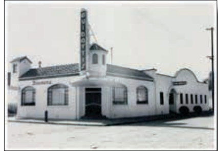
This 1948 photo shows Guidotti's Restaurant, built on the site of the original Toscano Hotel.
